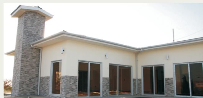
Wall Tile and Cement Board
