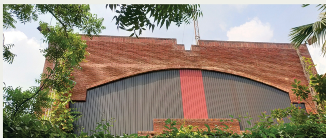
Exposed Brick Cladding
