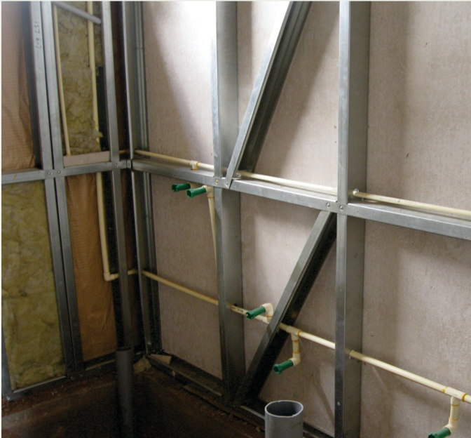
Arrangement of Pipe line for Various Services
