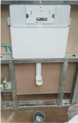
Wall / Floor mount WC Fixing Arrangement
