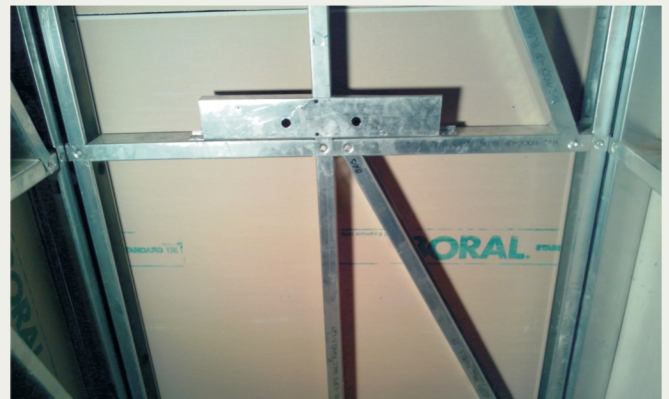
Wash Basin Fixing Arrangement
