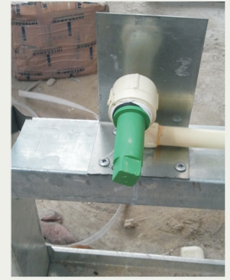
Tap Fixing Arrangement
