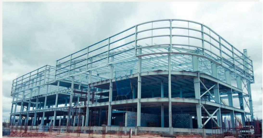
Typical Primary and Secondary Framing Systems
