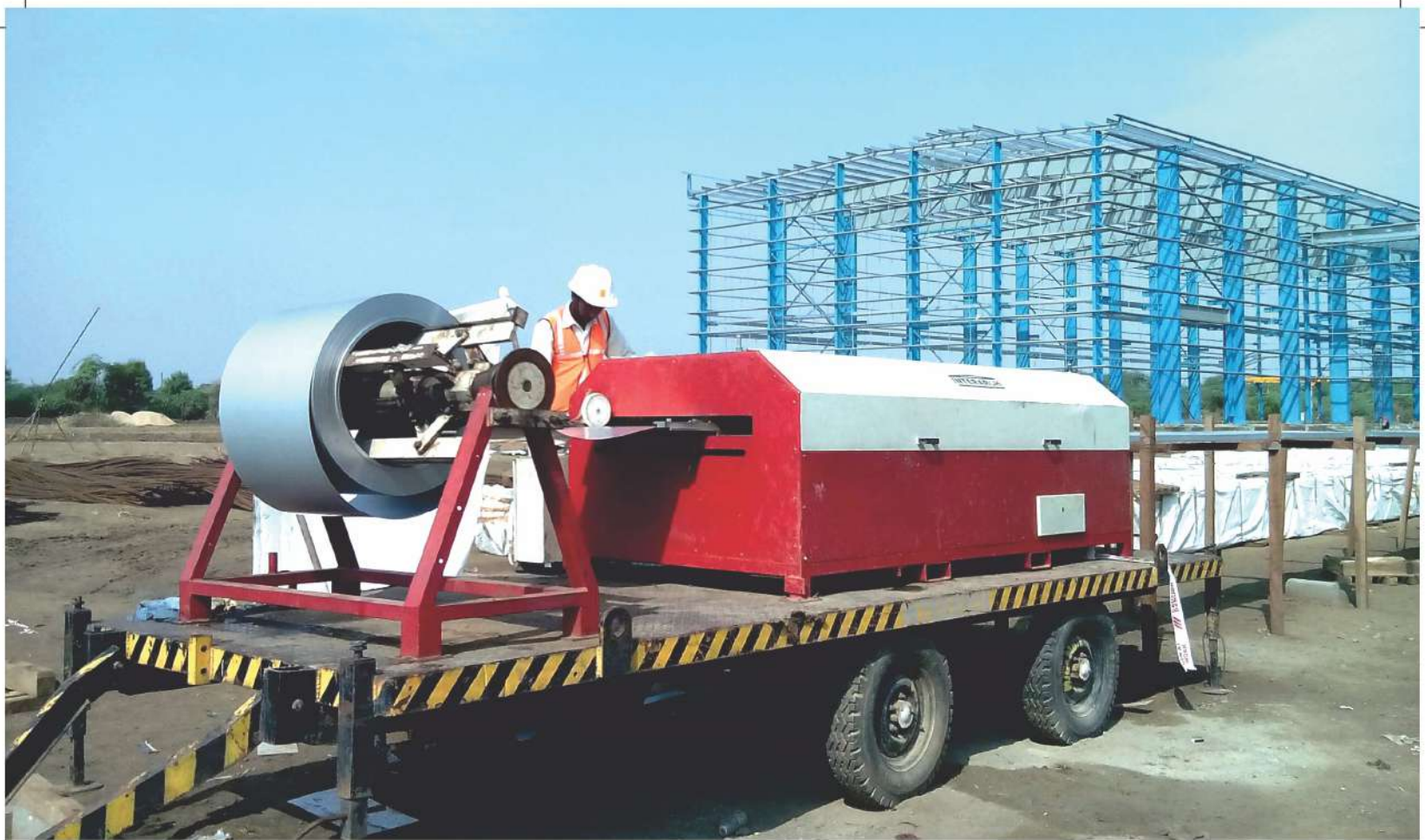
TRACDEK® SS-2000® On-site Roll Forming for Single Length Panels
