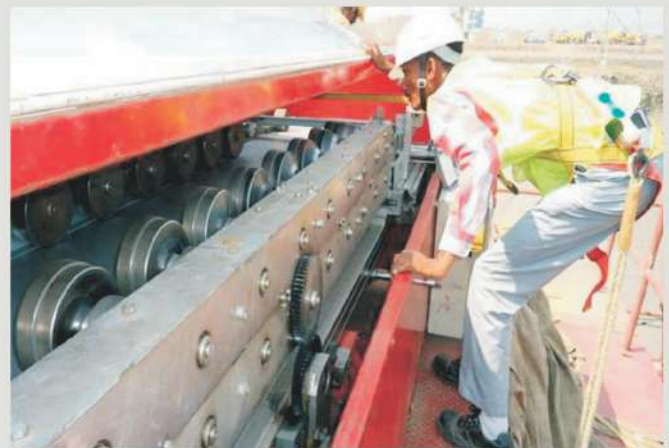
TRACDEK® SS-2000® On-Site Roll Forming
